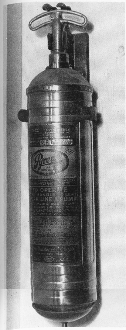
The Pyrene fire extinguisher which hangs on the wall at many points in Scovill City is made to squelch fires in oil or gasoline or around electrical equipment.
