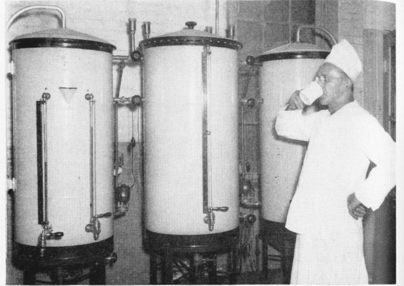
At the left, Ernest Goodreault, coffee specialist at the cafeteria kitchen on Silver Street, is putting a pound of coffee into the ledger at the top of one of the huge coffee urns. Above we see the complete battery of urns and tanks which keeps piping hot coffee flowing out to room cafeterias. It's the largest coffee unit in operation in New England and was built to order for Scovill use.
